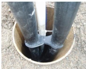
Figure 8. BHE7: U-pipe with spacers
