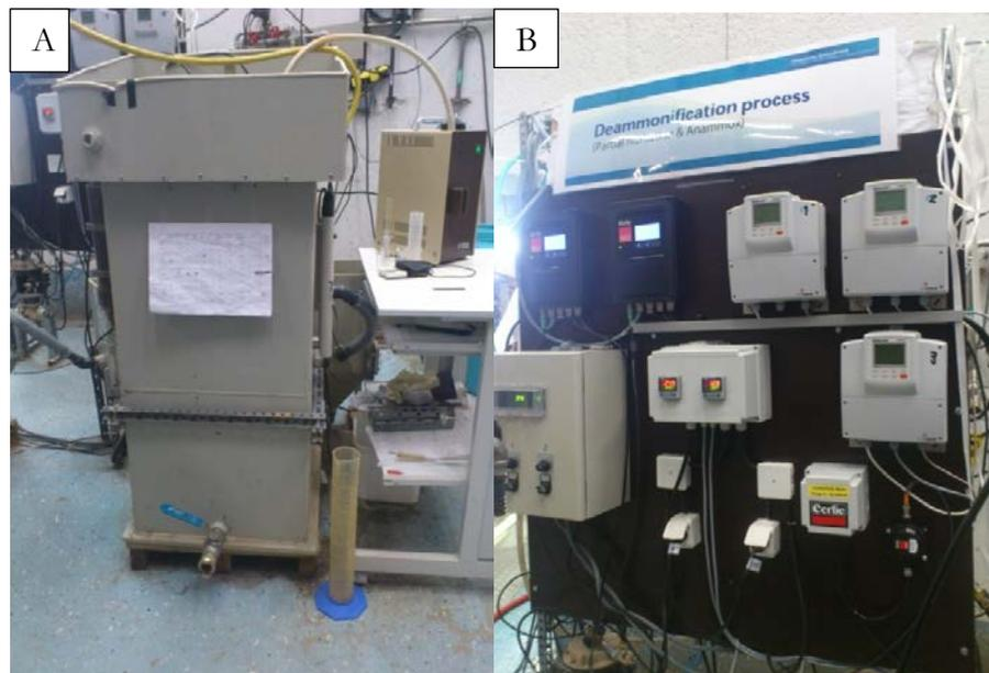
*Fig. 4: One stage deammonification system in pilot scale MBBR at Hammarby sjöstadverket: A) Moving bed biofilm reactor B) Control and monitoring panel.*
