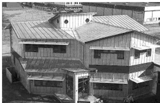
Figure 28. AB Halmstads Varmförzinknings office building, Halmstad, Sweden, illustrating large variations in building geometry and exposure conditions that need to be considered when calculating and predicting metal runoff rates. Reprinted with permission from AB Halmstads Varmförzinkning.
