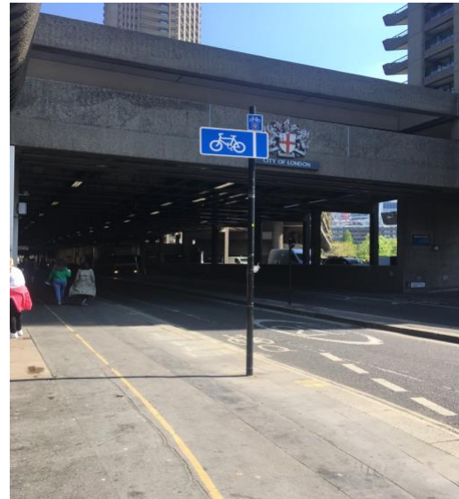
Figure A7.2. The figure shows the entrance to the tunnel where the Beech Street sensor is placed. Picture taken by Greta Gustafsson
