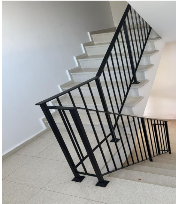
Figure 4.3. Designated emergency staircase of the dormitory.
