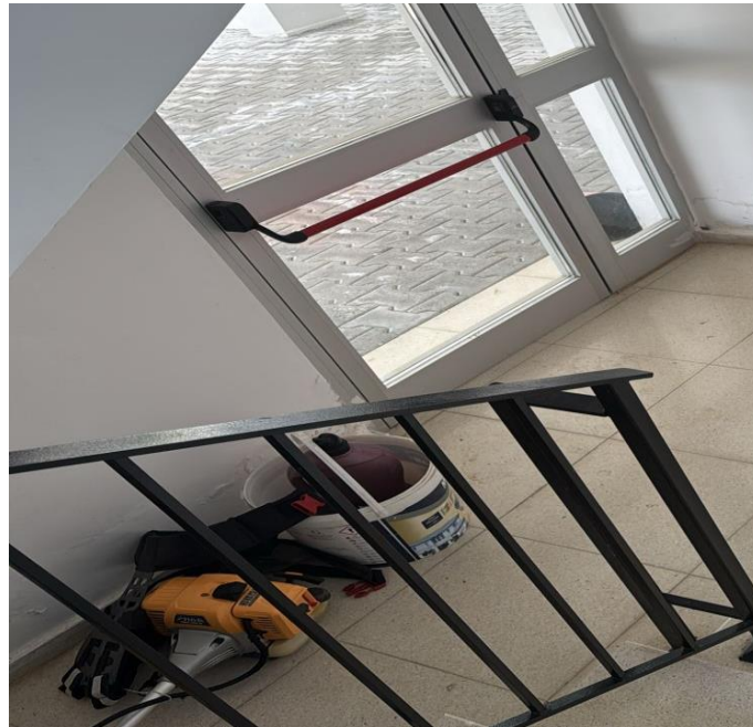
Figure 4.2. Emergency door of the dormitory and tools.
